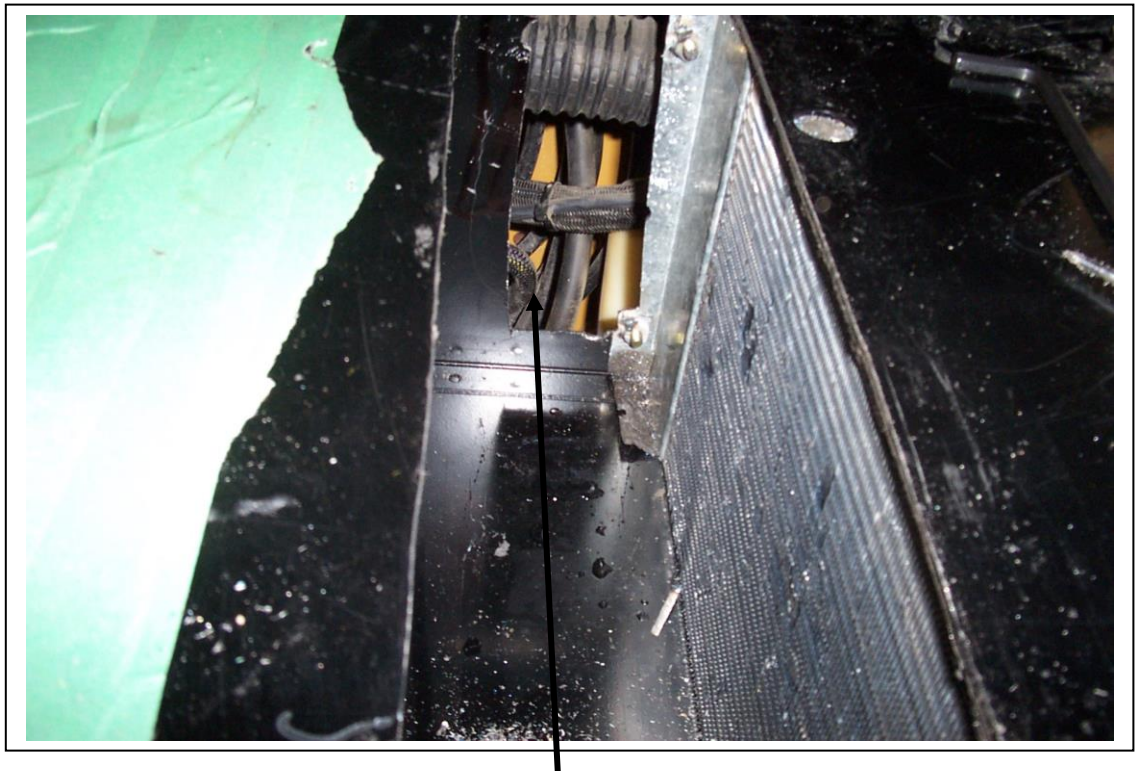
Hole cut out for expansion valve and hoses
